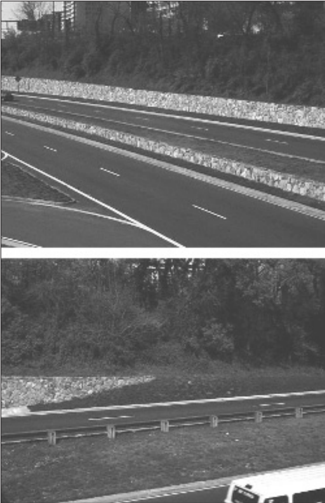
FIGURE 3-6 Special Aesthetic Barrier and Guardrail Meeting NCHRP Report 350 (17) Test Requirements
